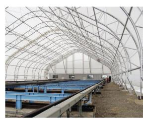
a truss arch building—created by a fabric, metal and hybrid building developer— which is 83 feet wide by 336 feet and 8 inches long.
